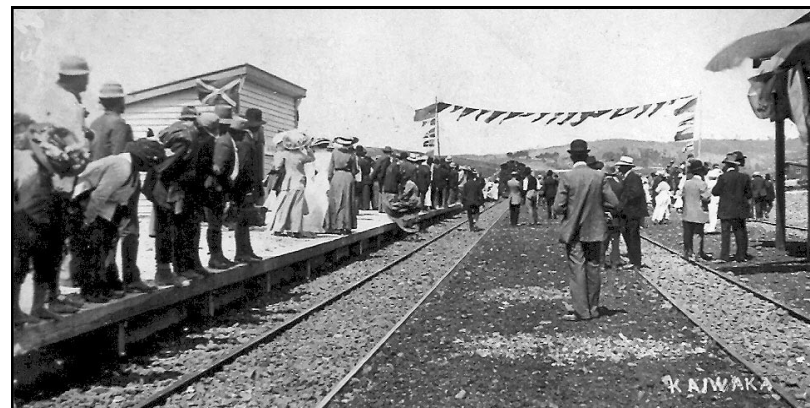
Kaiwaka Railway Station opening 18 March 1913
